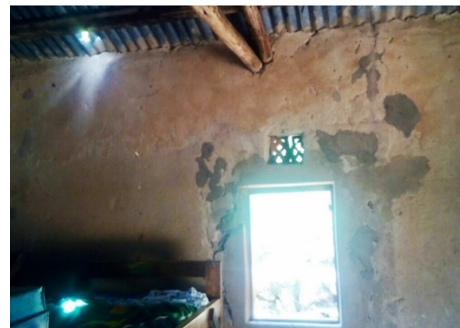
The dormitory is leaning rightward, not the camera! Obvious holes in the roof allow in rodents, bats, other pests, and rain!
