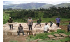
2005 - School drop-out youth working on foundation bricks
